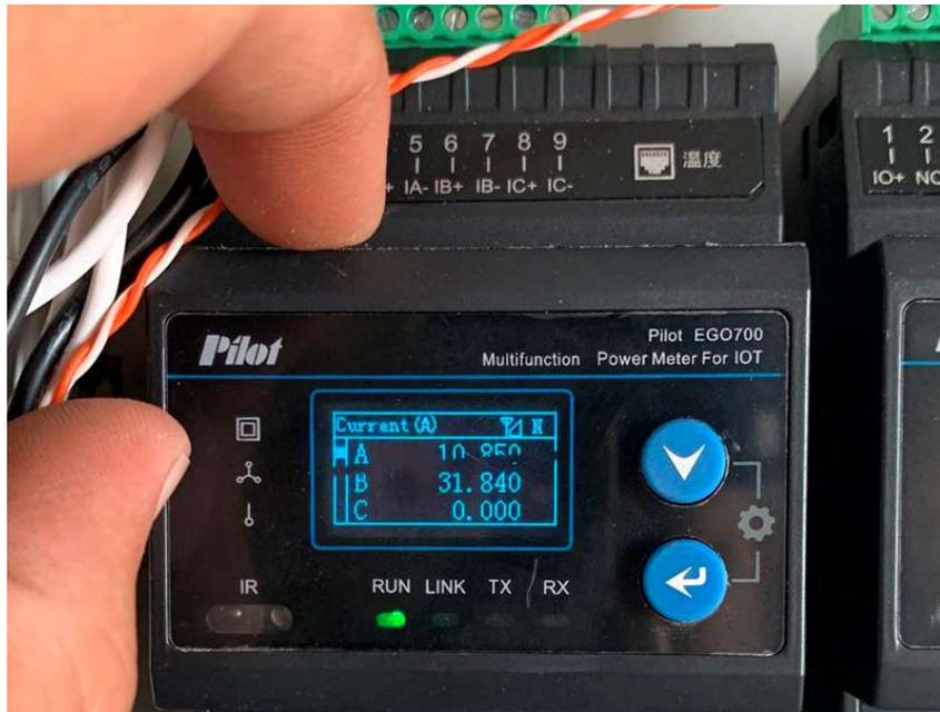
To implement the "field level", Pilot equipment was used as a PLC. The control equipment allows full control of the state of the diesel generator set, the city power supply of the AC, control of the DC power supply from batteries and solar panels.
